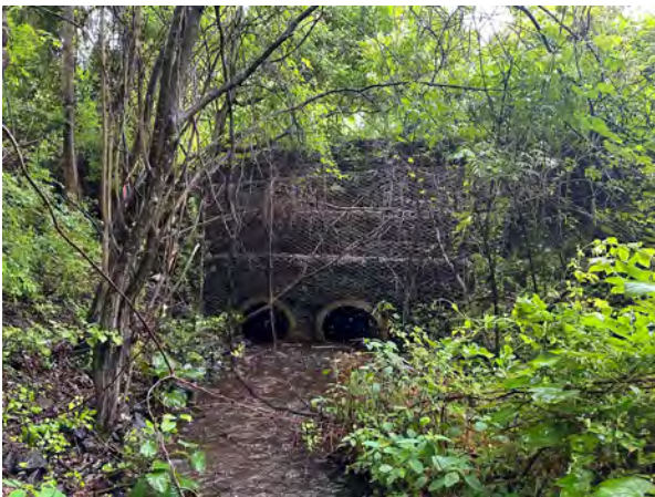
Reinforced concrete culverts channeling the stream beneath Memorial Drive
